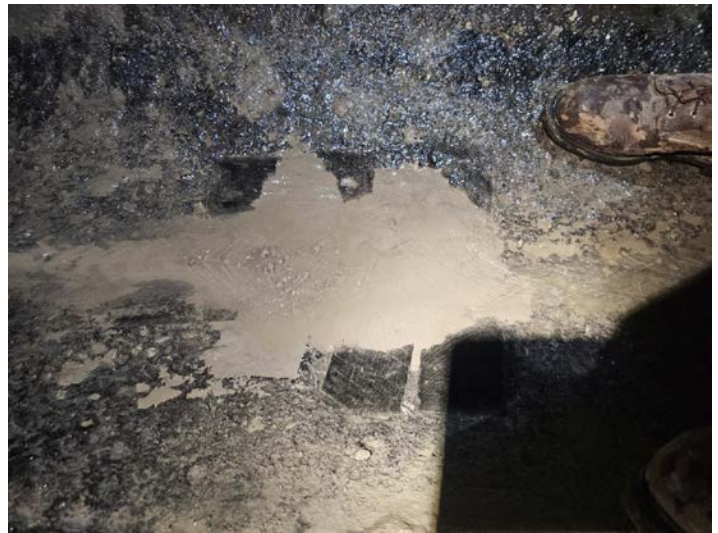
6C - Hole in the Eureka Sewer Interceptor
