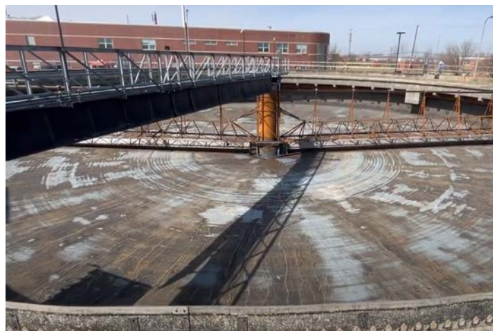
6C - Secondary Clarifier Towbro Arm Assembly
