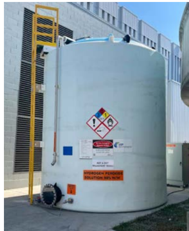
8D – Hydrogen Peroxide Storage Tank for Odor Control
