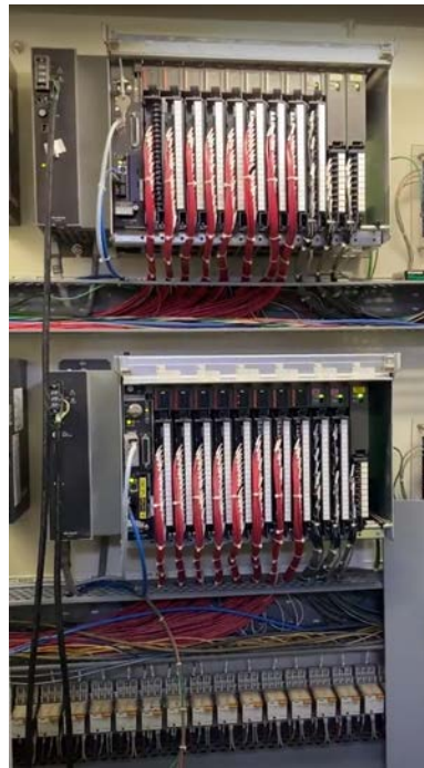
8B – Programmable Logic Controllers (PLC-5s) in Need of Replacement
