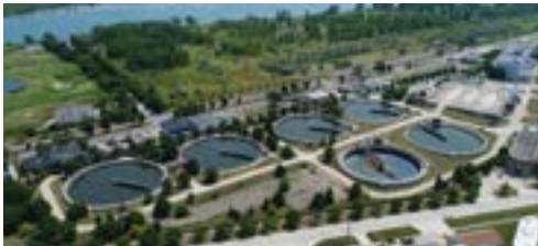
Downriver Utility Wastewater Authority 25605 Northline Road Taylor, MI 48180
