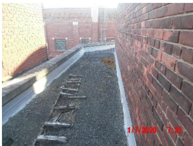
View of Lower Hallway Roof Section
