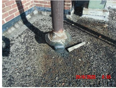
View of Roof Vent Sealant (Silver/Black)
