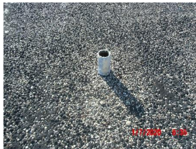
View of Typical Lead Roof Vent
