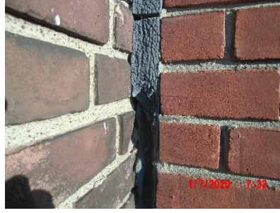
View of Expansion Joint w/Foam (Gray)
