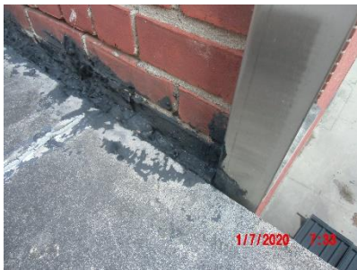
Additional View of Expansion Joint w/Foam
