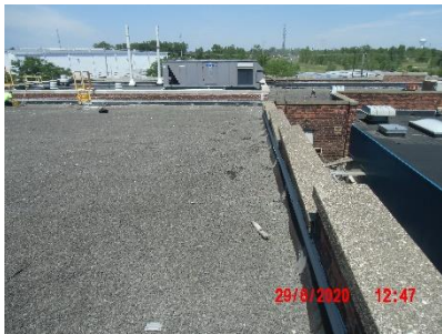
View of Section T.T. Coping and Sealant
