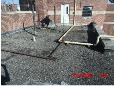
View of Typical Roof Vents
